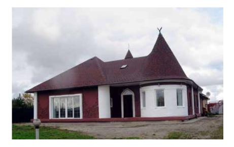
**Figure 40.** The first residential building in Europe printed with a 3D construction printer. Yaroslavl (Russia). Source: AMT-SPETSAVIA Group (Russia) – <u>www.specavia.pro</u>, CC BY-SA 4.0, <u>https://commons.wikimedia.org/w/index.php?curid=74334750</u>.
